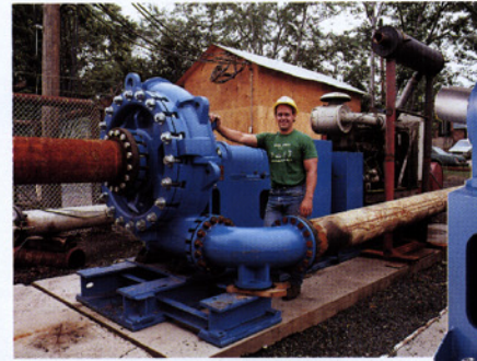
Portable diesel driven 5500 pumping gravel.
